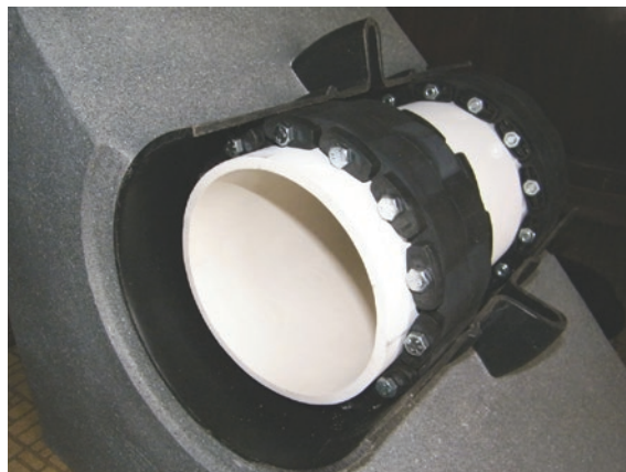
Cut-away view of Infinity® wall sleeve & Innerlynx®
