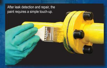
\*\*Two coats of paint recommended with coating thickness 1.4 - 2.2 mils when dry. Dry time 4 hours between coats.
