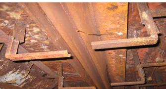
Combustion Engineering (CE) COR-TEN expansion joint - installed 1976
